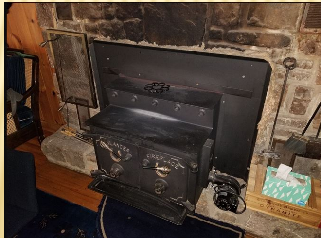
Woodstoves vented into unsafe chimneys
