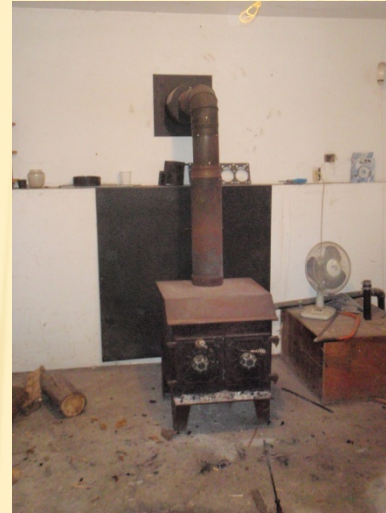
Woodstoves vented into unsafe chimneys
